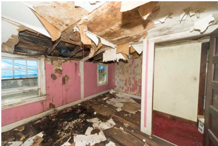
Water damage: Top: Apt LR | Bottom: Apt BR
