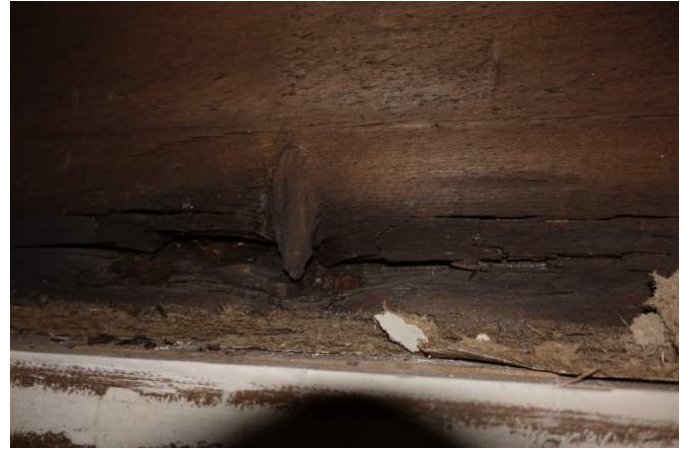
Figure 40 Insect and/or water damage to joist
