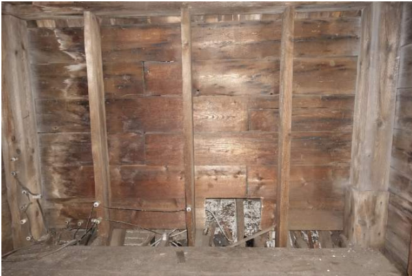
Figure 55 Inside the attic space above the entry and below the bell tower. Each corner is a 6" x6" post that travels through the framed assembly. This is looking south; you can see the ceiling of the Sanctuary beyond
