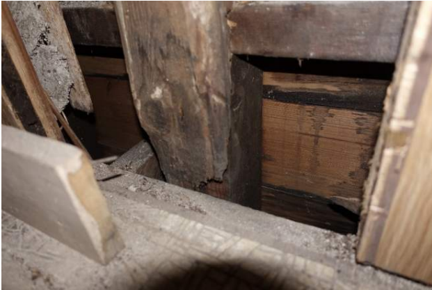
Figure 13 First view of base of post that supports eastern truss on north Sanctuary wall. This prompted us to expand the probe. The post has been cut and a repair using 2x6 has been inserted.
