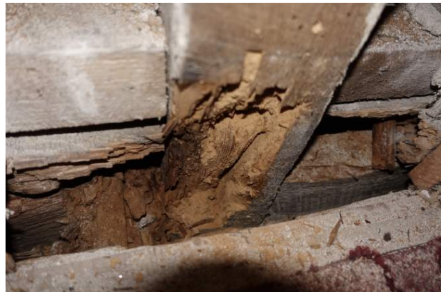
Figure 11 Base of western post that supports the truss on north Sanctuary wall was highly damaged by insects.
