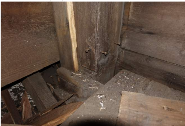
Figure 56 Close up of post just above the 2 nd floor level, where a butt joint that was hidden behind two boards nailed to the post is now visible. This is a hinge point in the column assembly.
