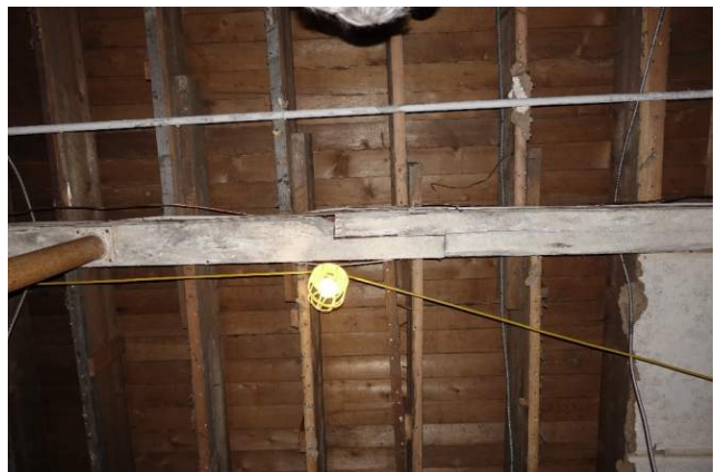
Figure 30 View looking up at half lap joint
