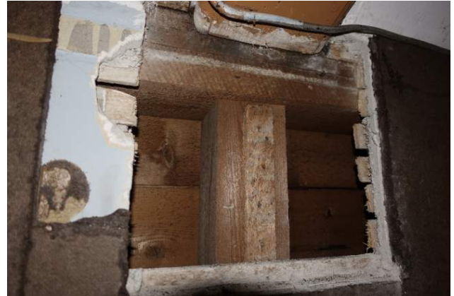
Figure 10 top of western truss on north wall of Sanctuary- wood is dry
