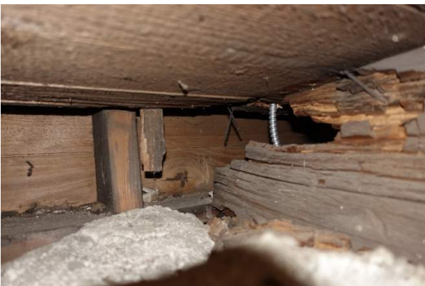
Figure 27 Another view of a fully rotted out joist, the wall framing visible here is the repair wood inserted along the north wall
