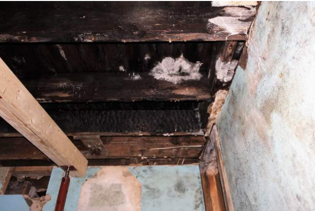
Figure 39 another view of burned joists
