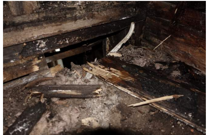
Figure 52 This is close up of the corner where you can see through the wall. The concern is if this part of the wall is this damaged, the header over the Apse needs to be observed for intactness
