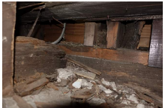
Figure 42 This is view between two joist bays in the Narthex. The rebuilt wall is visible beyond and the end of the joist is fully rotted away. The edge of wood visible at the far left of the picture is a sister joist
