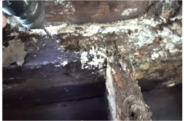
Figure 22 West end of 1939 addition top of wall with extensive rot
