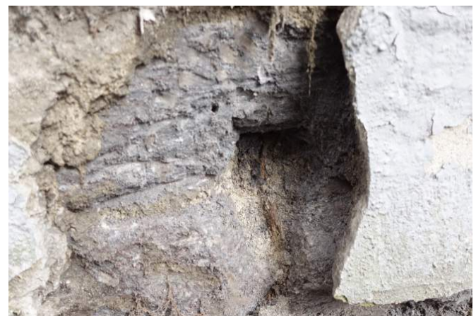
Figure 54 A close up of the wall indicates the grey loose, wet, and sandy material may be coming from this grey colored stone. The Church in town is built of a very similar stone.
