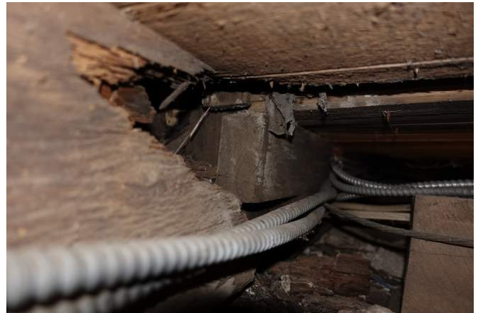
Figure 41 Joist end along north wall-possibly water or insect damage, or both. This is above the wood header between the main Sanctuary and the Narthex. The wood visible beyond are the Narthex joists
