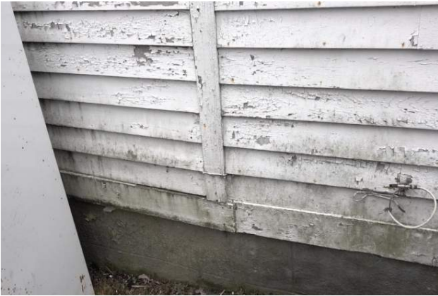
Figure 19 Transition between 1886 and 1890's where base of north wall had deterioration behind sheathing.
