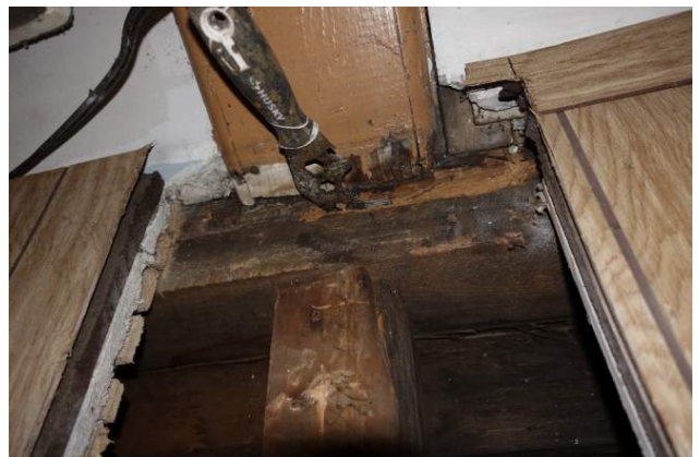
Figure 12 Top of eastern truss on north Sanctuary wall with significant insect and moisture damage
