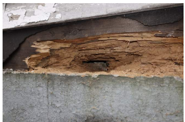
Figure 18 The rot in the base plate traveled through to the inside of the basement.
