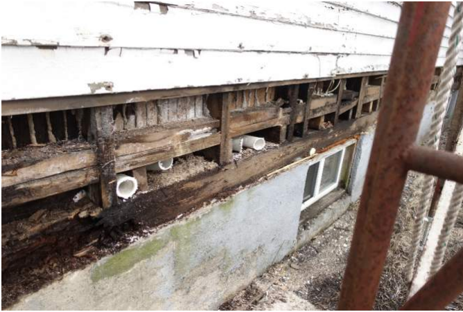
Figure 1 – Lower zone of deteriorated south wall of the Sanctuary
