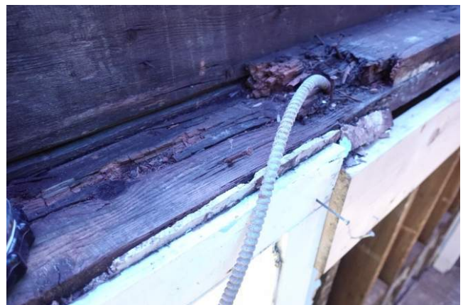
Figure 23 Top of 1886 south wall (west wing) with joists already removed.
