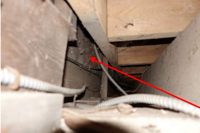
Figure 43 This is a view of the raised floor built on top of original joists under the Apse. The arrow points to wall framing that appears to have no bearing. This needs further evaluation
