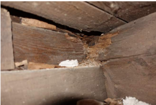
Figure 26 Close up of highly deteriorated joist where it bears on the base plate of the north wall.
