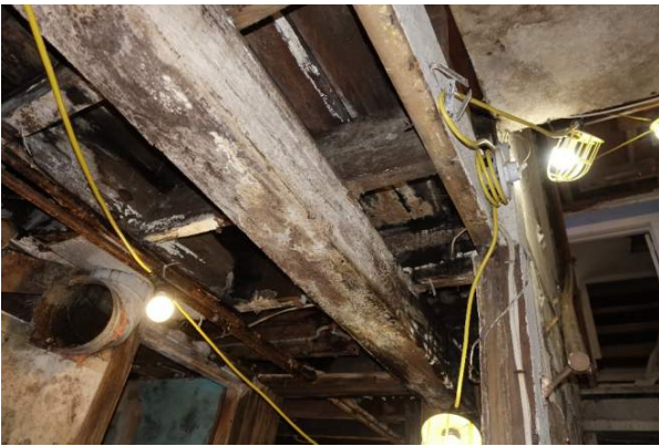
Figure 32 This is the 3 rd wood girder, south of the staircase that starts at the west 1886 foundation wall and ends on the chimney masonry pier
