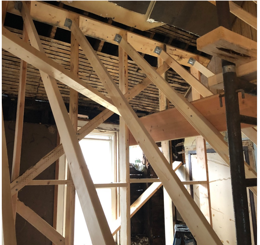
Interior shoring and exterior protection of south sanctuary wall | 10.23.20
