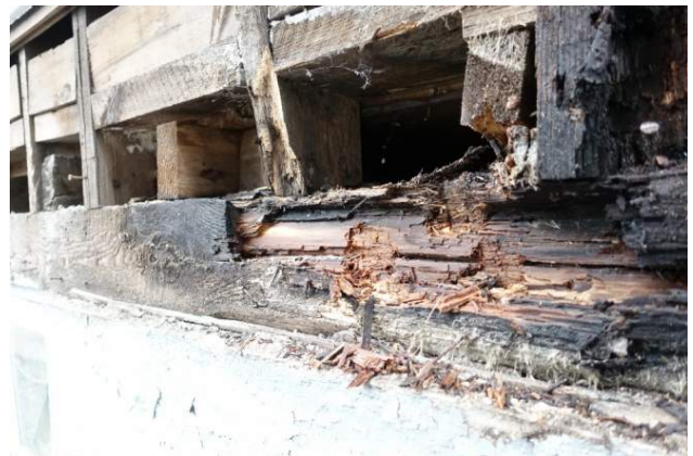
Figure 5 Close up of highly deteriorated base of south Sanctuary wall
