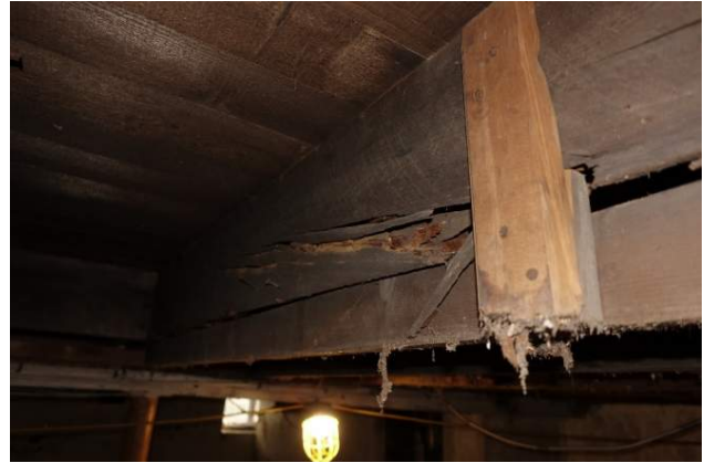
Figure 34 This fully failed and rotted joist is the northwest trimmer for this headered condition
