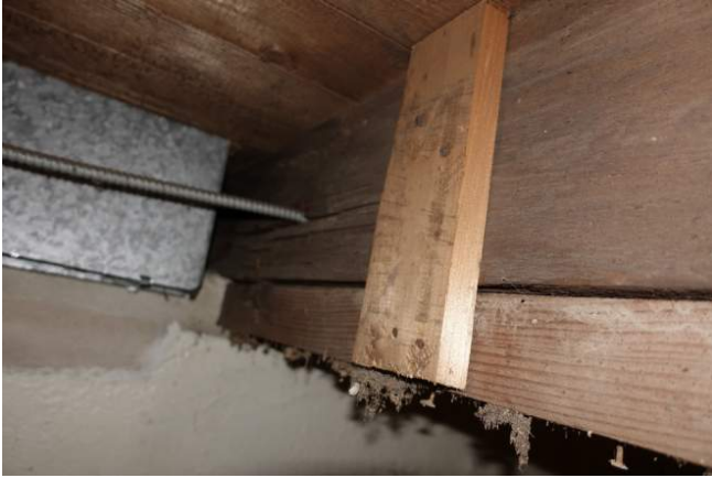
Figure 37 blocking installed in much of the main Sanctuary, possibly to align with the bigger joists in the kitchen when the ceiling was installed. Prior to ceiling panels being removed, this blocking gave the impression the 6" x 6" wood girder was smaller than it is. The joists are more commonly 7 1/2" high
