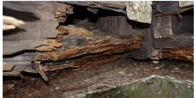
Figure 16 Close up of Narthex deteriorated base plate
