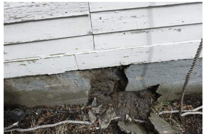
Figure 53 Foundation wall disaggregating behind the stucco finish
