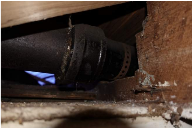
Figure 50 Cut joists below the bathroom and its cast iron bathtub. At last three were observed to be cut to the point the joists cannot hold weight
