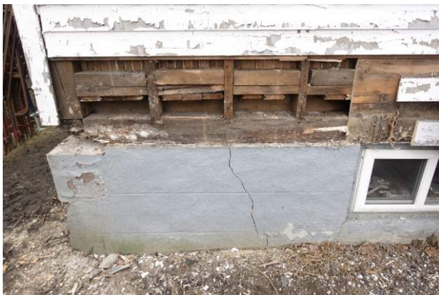
Figure 3 Overall view of the south wall of Sanctuary wall exposed. The damage is contained to the west corner. Note the crack in the foundation wall that should be further evaluated.
