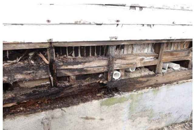
Figure 6 Transition zone where highly deteriorated wood becomes dry to the right side of photo, left side of photo is west end of Sanctuary with extensive rot.
