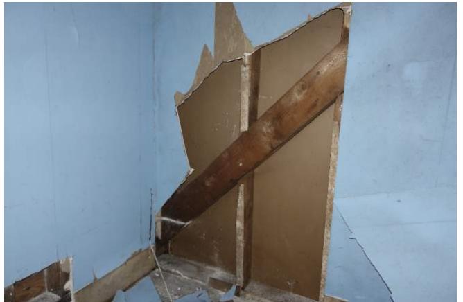
Figure 47 Close up of double roof rafter passing through the wall and studs built to it.
