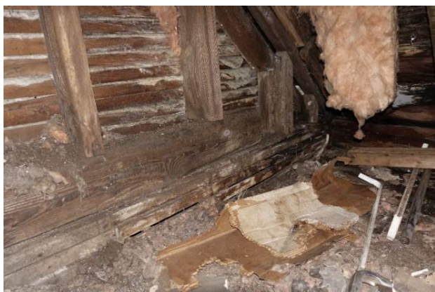
Figure 51 Inside closet toe h south of the chimney at the 2 nd floor. You can see the plaster wall that is the interior of the Sanctuary. There is an embedded double plate that framed the gable end of the sanctuary. You can see the wood is deteriorated.
