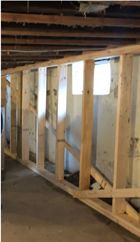
Interior shoring and exterior protection of south sanctuary wall | 10.23.20
