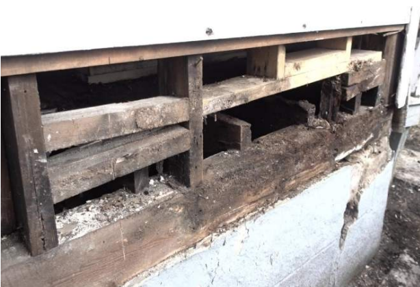
Figure 21 Part of southwest corner of building at west wing. Combination of rotted and dry wood. You can see the two replaced studs.
