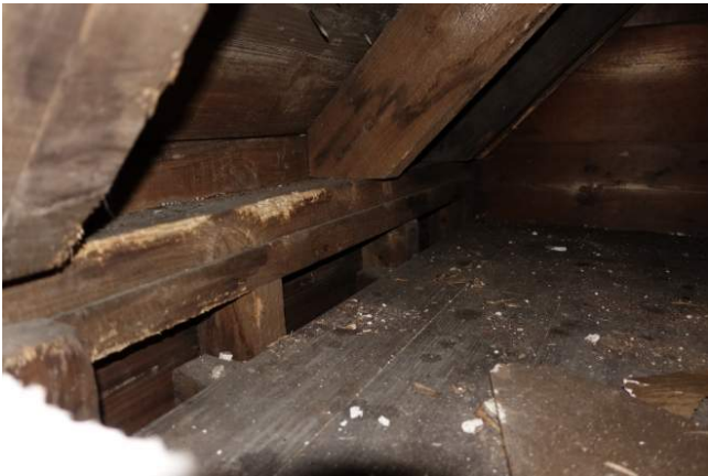
Figure 44 View of the balloon style framing used on the north half of the 1890's addition. You can see the 2 nd floor joists below the floorboards about three inches lower than the bottom side of the double top plate of the wall and rafters bearing on the top side.
