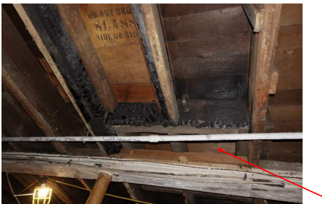
Figure 33 Location of earlier hole in the Sanctuary floor about 24' x 26" wide – two spanning joists are headered off at the opening. At this location, 30" of the 6" x 6" wood girder had been cut out. Due to this cutout, the 6" x 6" girder is cantilevering off the post to the east about 2'-0"
