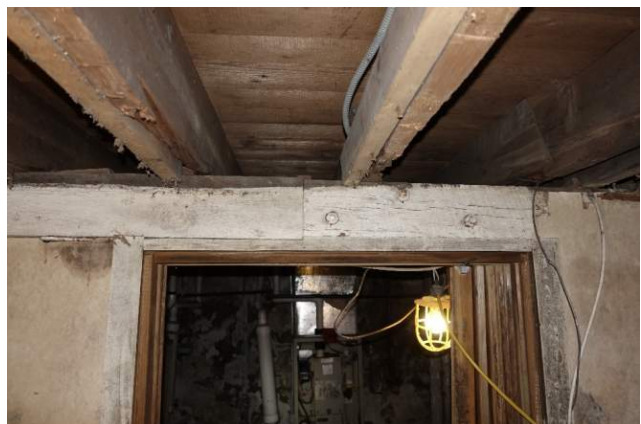
Figure 29 This is a view of the half lapped joint in the center 6x6 wood girder located over the doorway into the kitchen.
