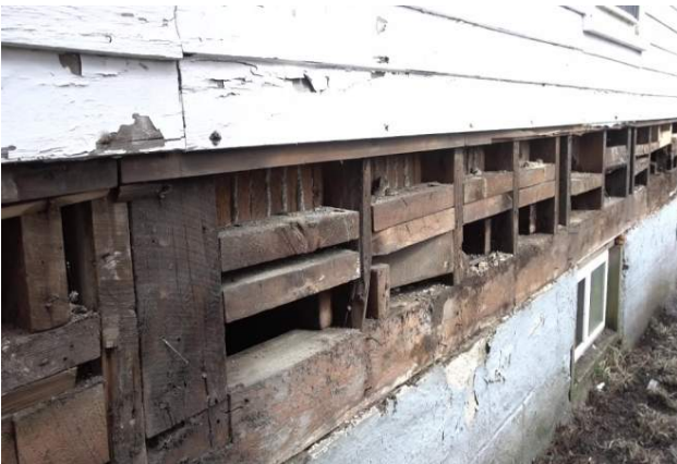
Figure 20 Overall view of southwest corner of south wall (west wing). The 6x6 post in the foreground is the end of the original 1886 building. The left corner shows the beginning of the 1939 addition
