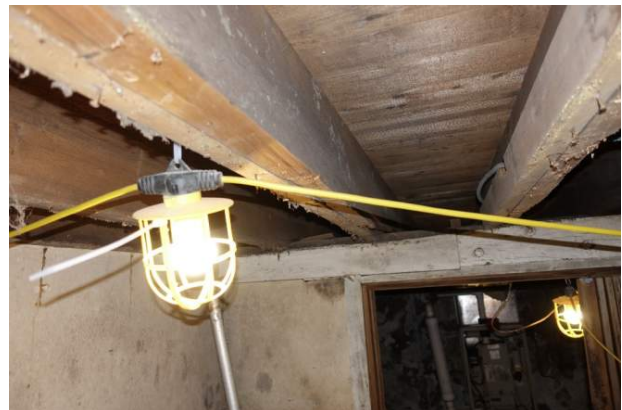
Figure 36 Bottom of joist was cut crudely along its bottom, possibly because it was too low for the ceiling
