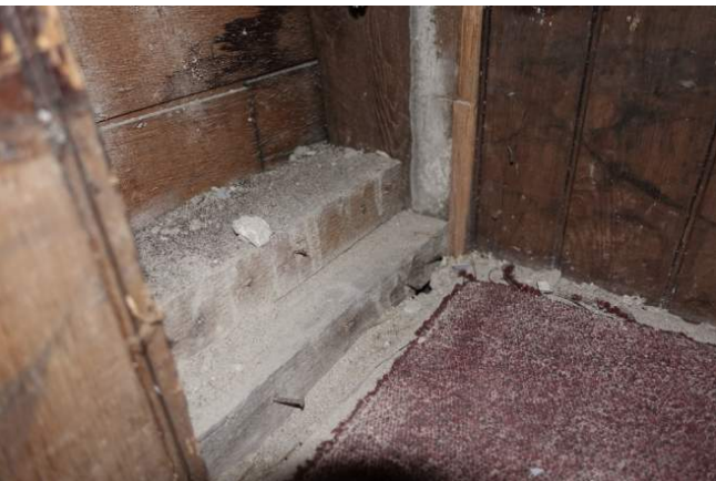
Figure 9 Base of northwest corner of Sanctuary- wood is dry. We only observed the inner face of the 6x6 post. The back side of the wall has exterior sheathing visible as this was an exterior wall originally.
