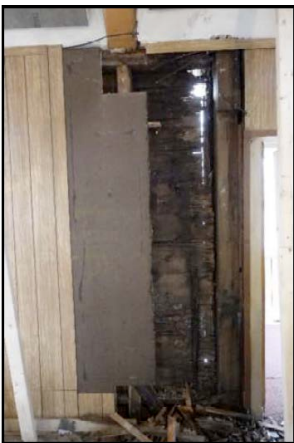
Figure 14 Larger probe performed to uncover 2 fully rotted studs that crumbled upon removal of plaster. Note daylight coming through the wall.
