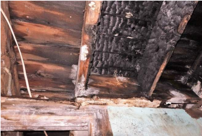
Figure 38 Burned joists
