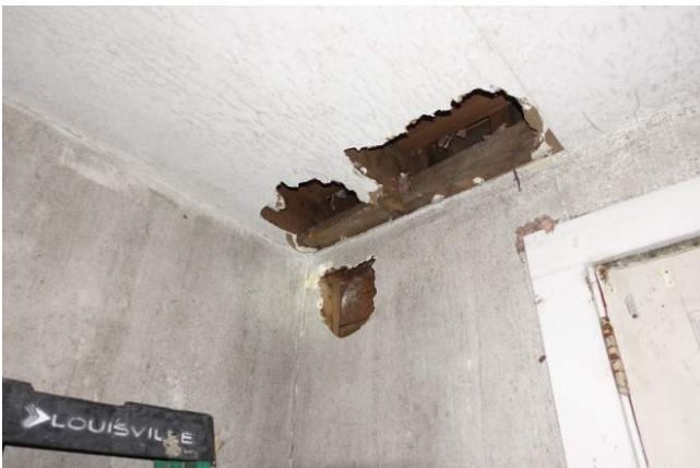
Figure 45 View from the 1st floor ceiling along the north wall of the west extension. The wood between the joists is just a nailer for the ceiling. The joists are nailed to the side of the studs
