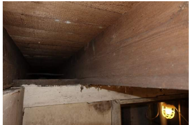
Figure 35 Kitchen joist that is notched to go over 6" x 6" wood girder because it is 8 1/2" high
