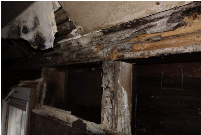
Figure 2 The inside of the south wall of the Sanctuary exposing the top plate and studs below
