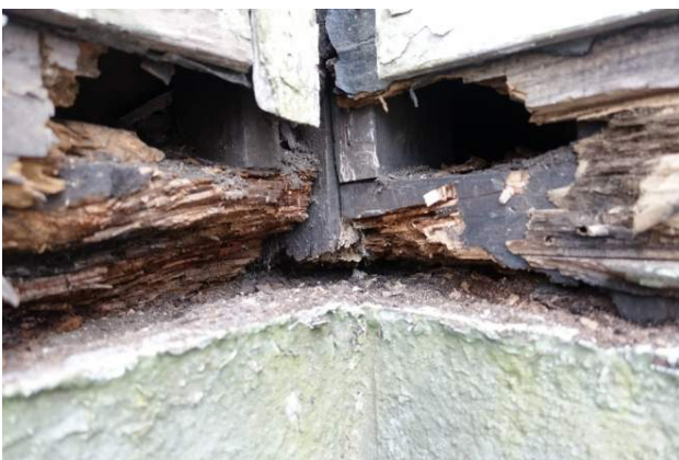
Figure 15 View of exterior corner between Narthex and north wall of Sanctuary. Note the degree of rot in the base plates here.
