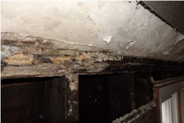
Figure 7 Top of south side of Sanctuary from inside- note saturation and mold
