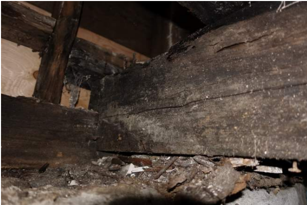
Figure 25 View of a joist notched to bear on top of 6x6 base plate. The bearing end is often in very poor condition.
