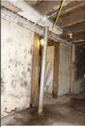
Figure 31 View of the 2 nd wood girder that is south of the main wood girder. The door opening visible is to the kitchen. The girder starts at the west 1886 foundation wall and ends at the post visible in this photo
