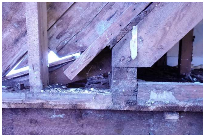
Figure 48 Western end south dormer and its connection to a triple plate that bears on 2 nd floor joists. Beyond to the left is the 2x4 extension of the roof rafter that travels another 4 feet to the top plate of the south exterior wall.
