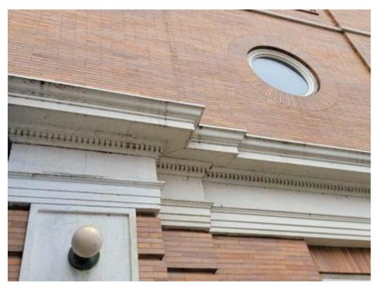
Detail photo of the lower soffit that is need of painting.
