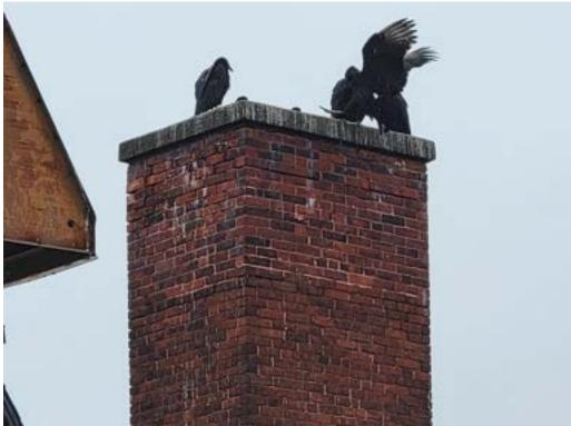
Another part of this project would be the repointing and capping of an unused chimney. These photos show the top of the chimney where the mortar has failed and the repointing needs to be done to the brick.
