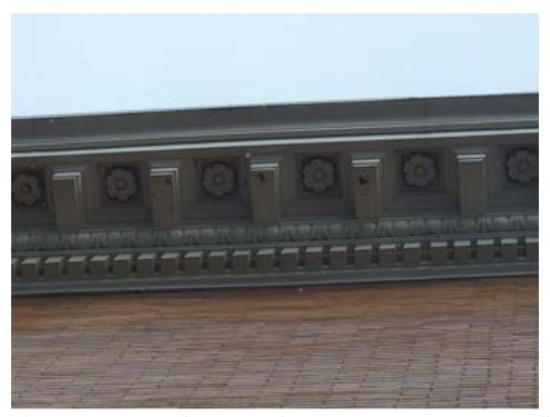
Detail photos (photo above and below) showing the failing paint on the upper decorative soffit that is in need of repainting as part of this project. With exposed metal from the failing paint, the soffit is prone to rust and deterioration.
