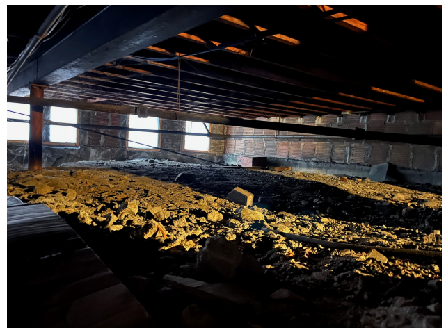
Foundation under book stacks with light showing through the floor boards in the 1930 addition in the back. Photo taken 11/26/23
