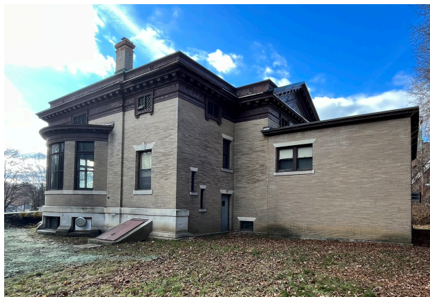
1930 addition showing separate piece without full foundation.
