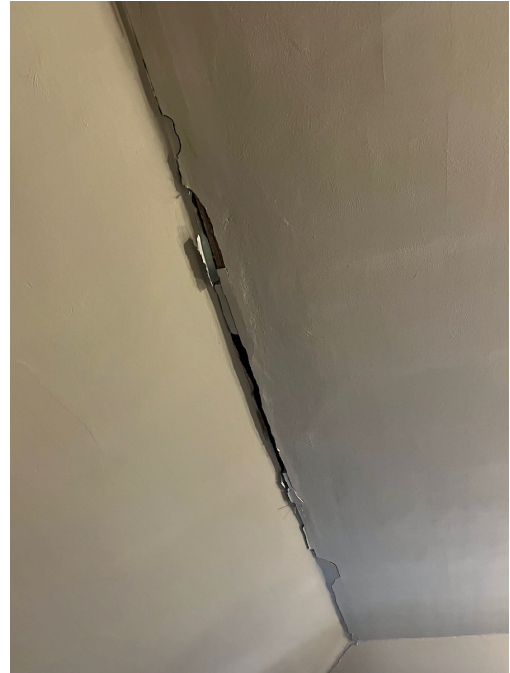
Plaster falling from second floor
