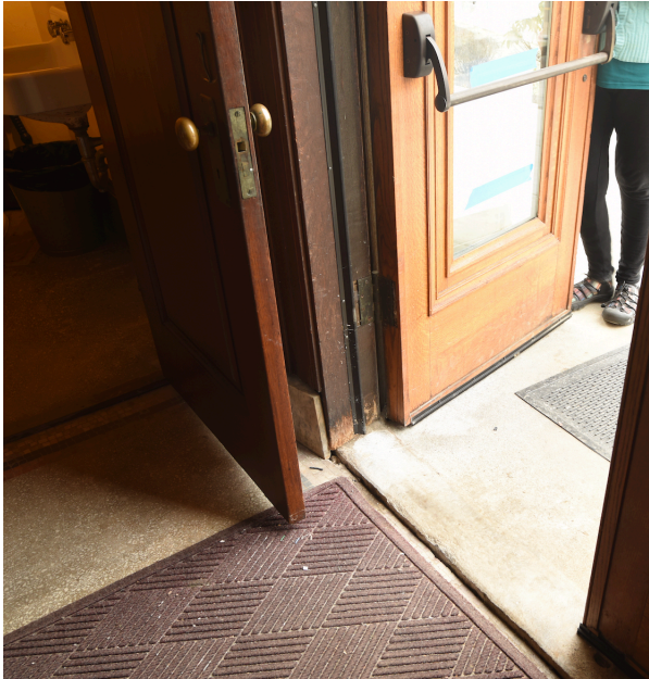
Front door and Bathroom door— cannot open bathroom door without impinging on people coming in.
