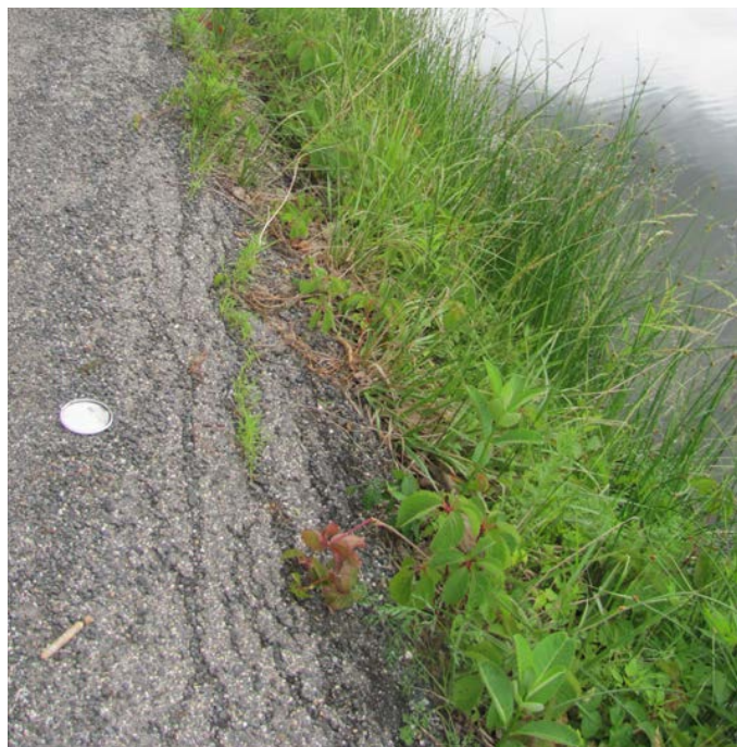
Road edge sloughing off into the lake, June 2015
