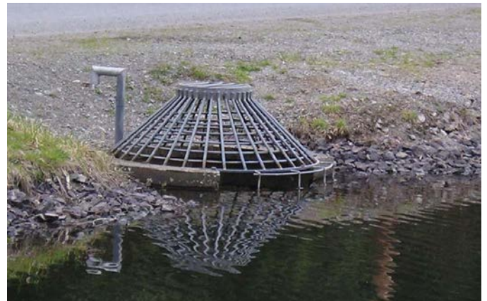
Example outlet control structure; Courtesy of Woodard & Curran
