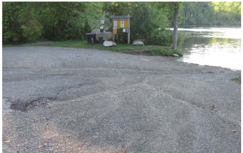
Launch point and erosion in parking area of boat launch, June 2015
