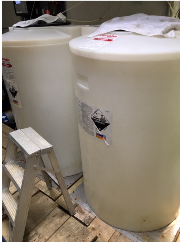
Chlorine disinfection storage tanks
