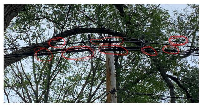
The circled areas are where the line had sustained damage in the past and needed repairs.
