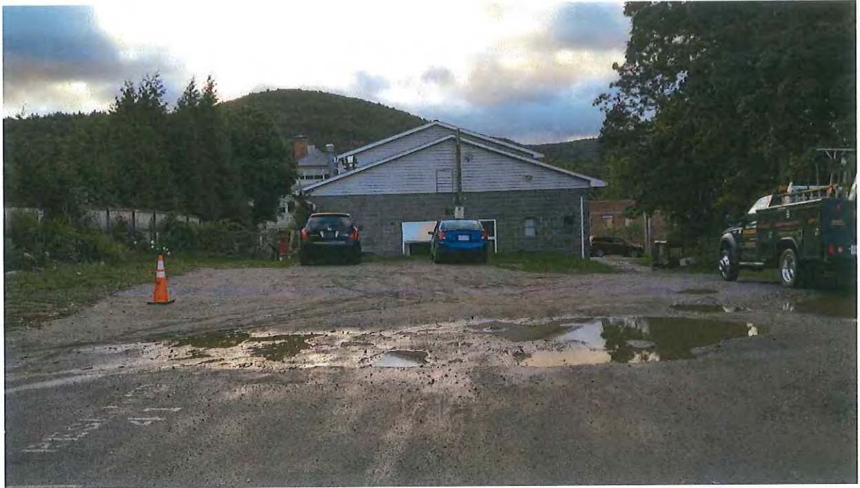
North Side of Building, Gravel Parking Area
