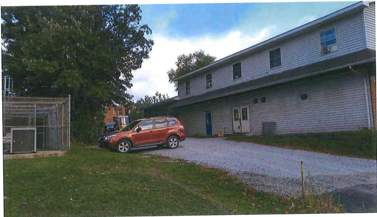
West Side of Building, Gravel Driveway
