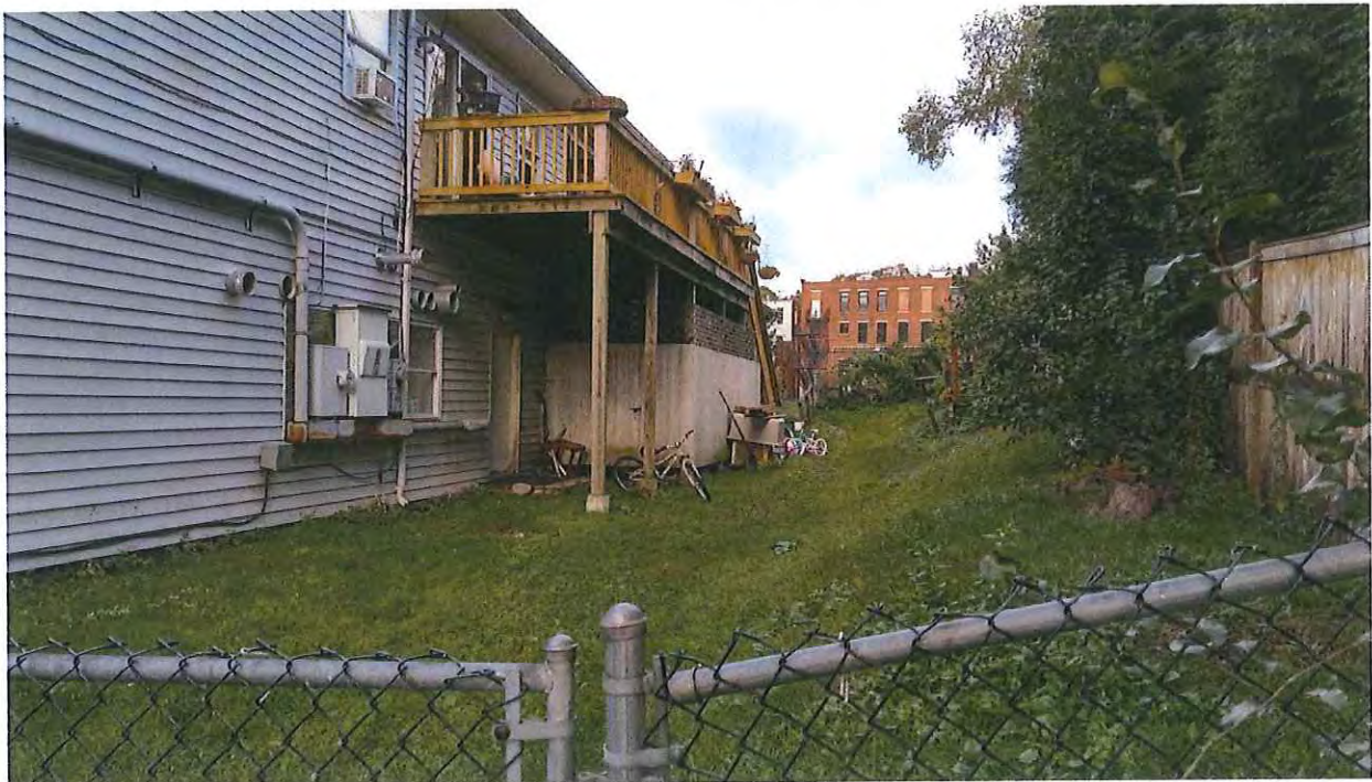
East Side of Building, lawn area and residential access
