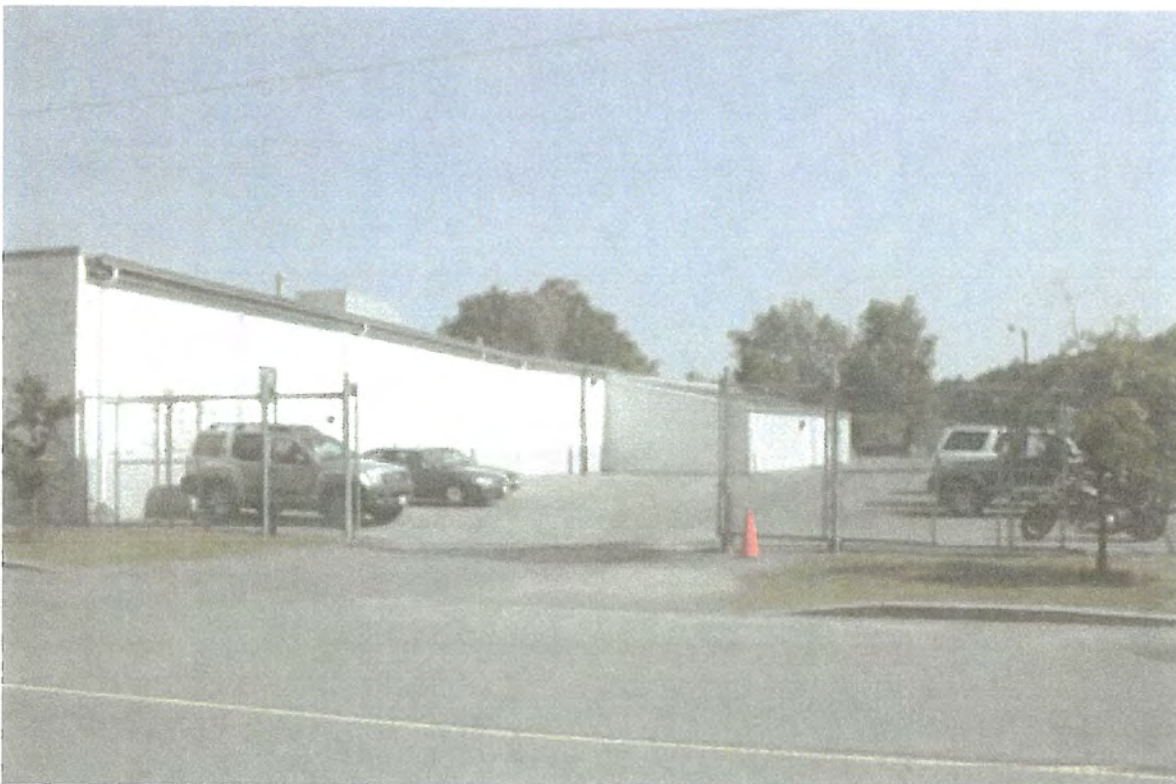
East side of building remaining untouched.
