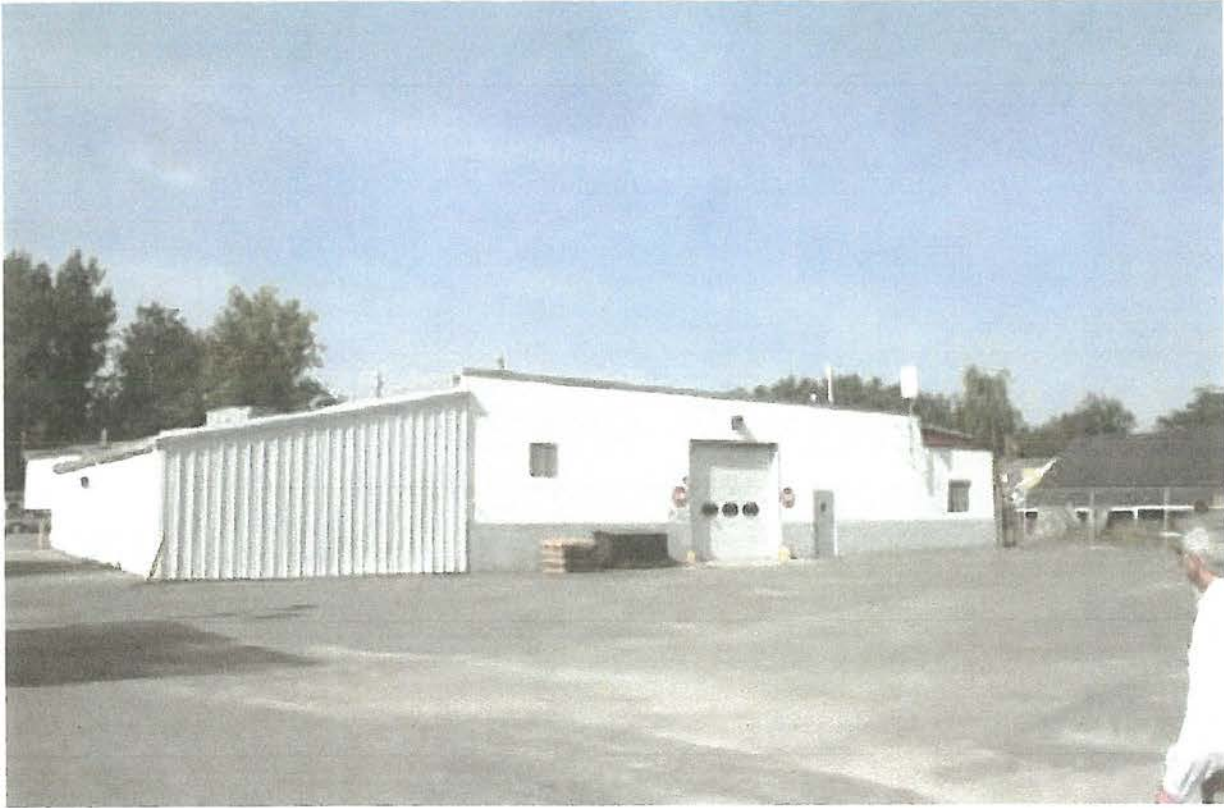
Rear of building. Overhead garage door to be framed in with double doors.
