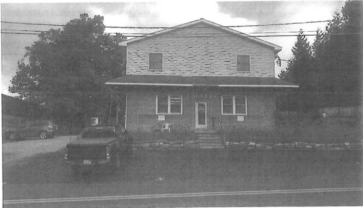
South Face of Building from School Street, existing paved parking area
