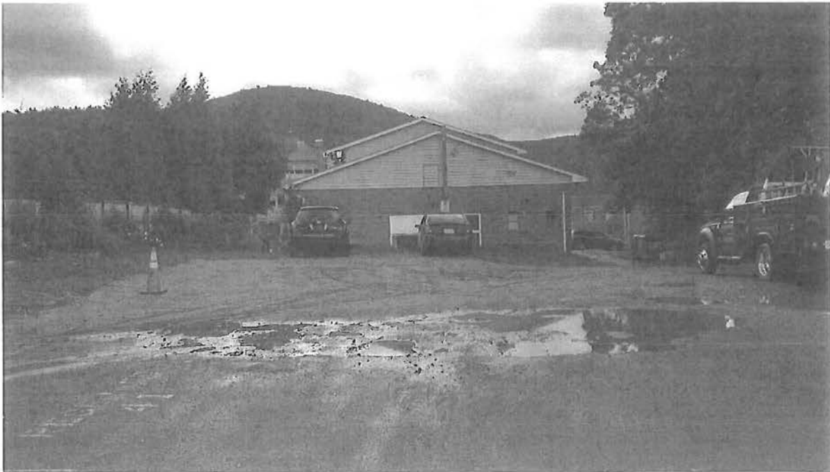
North Side of Building, Gravel Parking Area
