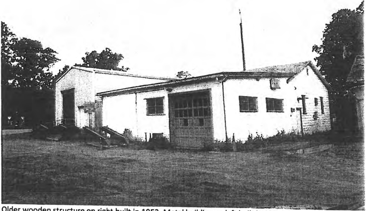
Older wooden structure on right built in 1952. Metal building on left built in 1988.
