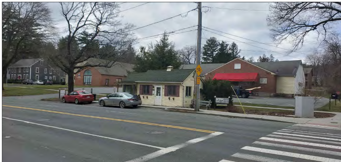
③ Existing East and North Elevations
